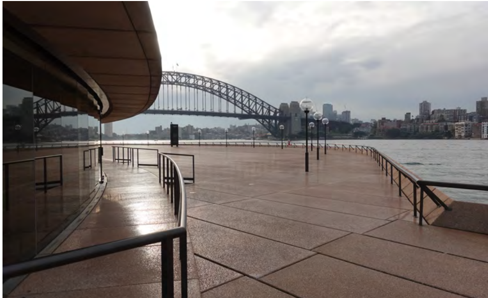
View 16 – from eastern extremity of Northern Broadwalk at northern end of Eastern Broadwalk, adjacent to Yallamundi Rooms
